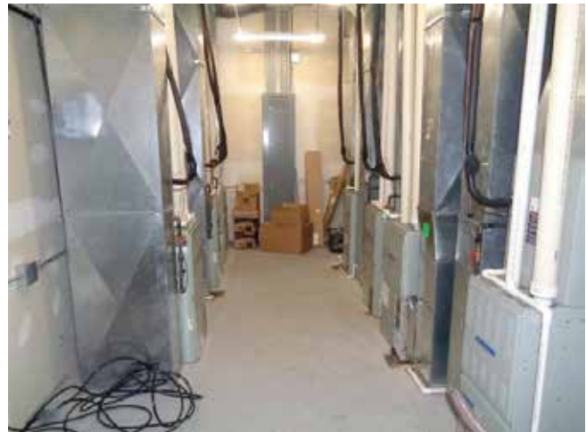
HVAC System Room
