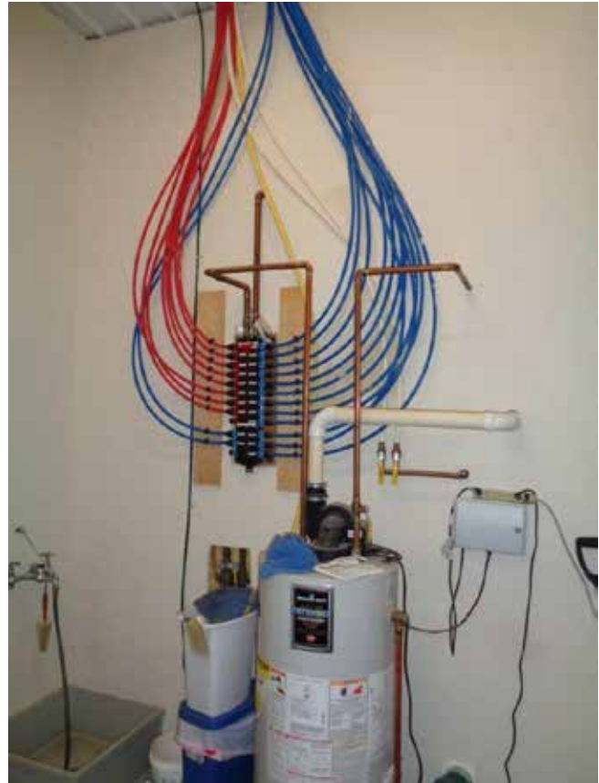
Water Manifold System
